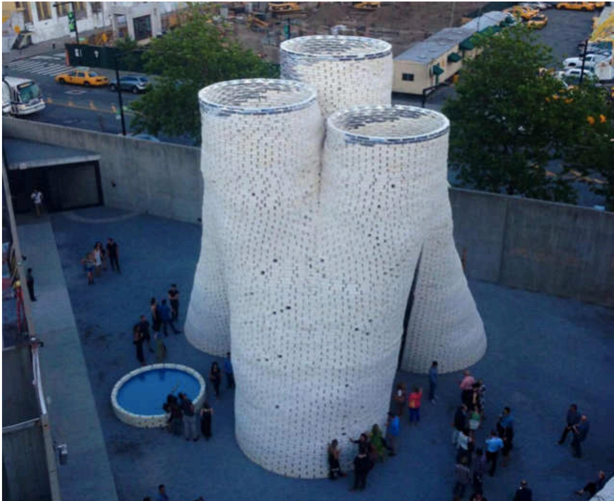
The Living project, constructed from blocks grown with mushroom mycelium. Photo: Cecil Barnes V
