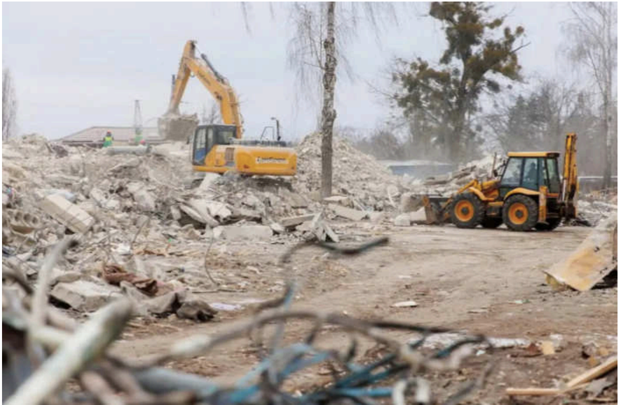
Equipment removes construction debris caused by Russian shelling. Gostomel. Photo: Neo-Eco
