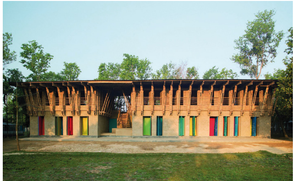
Abb. 7: Meti School Handmade, Rudrapur Bangladesch © ZRS Architekten Ingenieure
