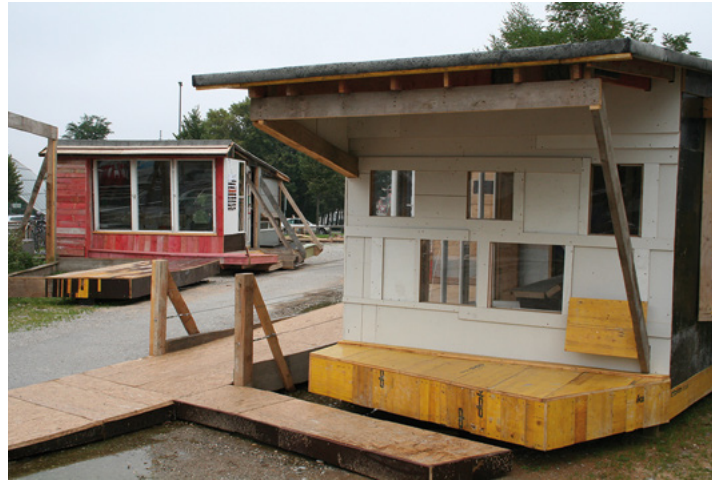
Fig. 22: Temporary structures, 2006, wooden slats, roofing felt, found materials © Folke Köbberling and Martin Kaltwasser
