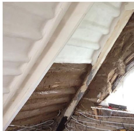
Fig. 19, 20: Multifunctional, multi-layered solution: Thatched roof plastered with clay on the inside © Elisabeth Endres
