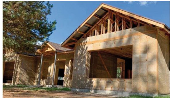
Fig. 16–18: Timber frame construction with hempcrete and hemp-lime infill in various construction phases © Hempire
