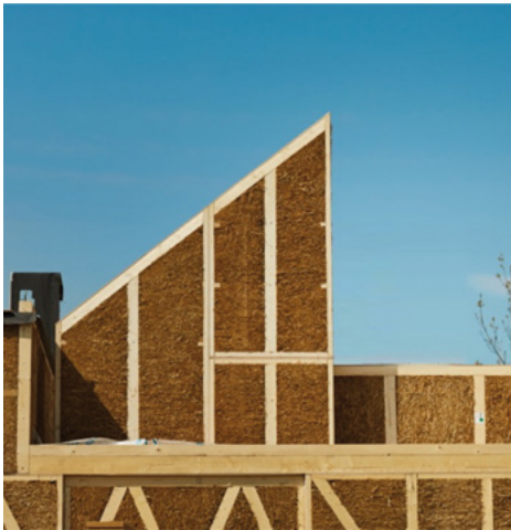
Fig. 21–23: Industrially prefabricated straw-insulated modules © Artem Ryzhkov, Life House Building
