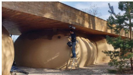
Fig. 14: Processing procedure with clay decorative plaster © Glinko
