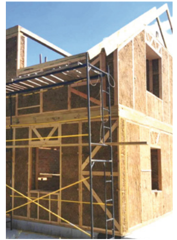
Fig. 18–20: Industrially prefabricated straw-insulated modules © Artem Ryzhkov, Life House Building
