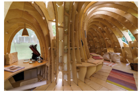
Fig. 10: Exterior and interior views of MY-CO SPACE. A curved interior made of plywood arches covered with mycelium © Wolfgang Günzel, tinyBE
