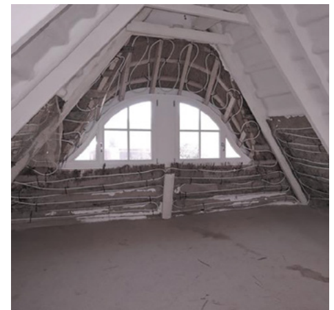
Fig. 19, 20: Multifunctional, multi-layered solution: Thatched roof plastered with clay on the inside © Elisabeth Endres
