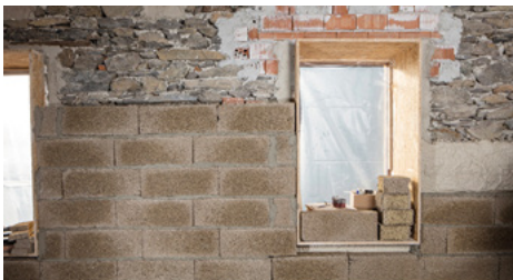
Fig. 22: Hanfstein interior insulation © www.hanfstein.eu
