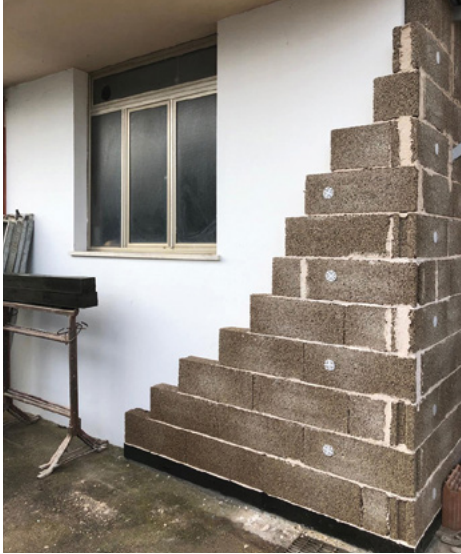
Fig. 20: Hemp blocks as external insulation © www.hanfstein.eu
