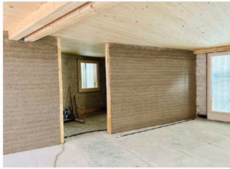
Fig. 23: Wall made of hempcrete © www.hanfstein.eu
