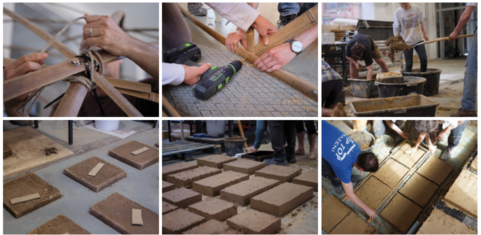
Fig. 10: Beehive © Natural Building Lab
