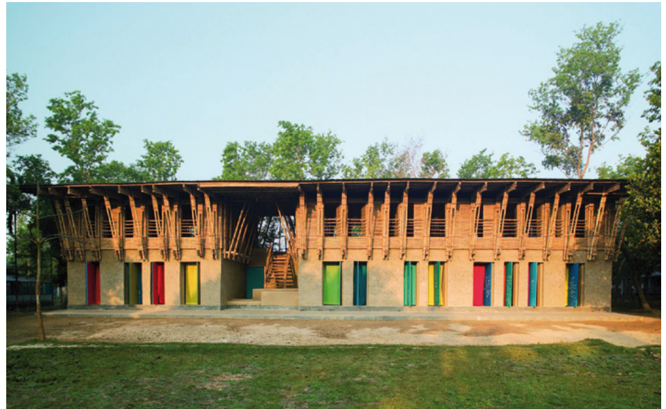
Fig. 7: Meti School Handmade, Rudrapur Bangladesh © ZRS Architects Engineers
