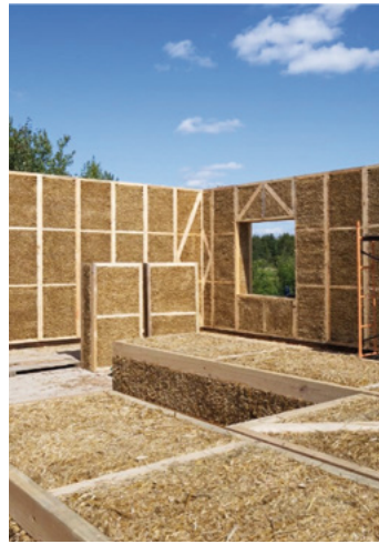
Fig. 18–20: Industrially prefabricated straw-insulated modules © Artem Ryzhkov, Life House Building
