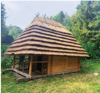
Fig. 22: Open-air museum in Lviv, stepped thatch covering, 40–60 cm thick reed walls
