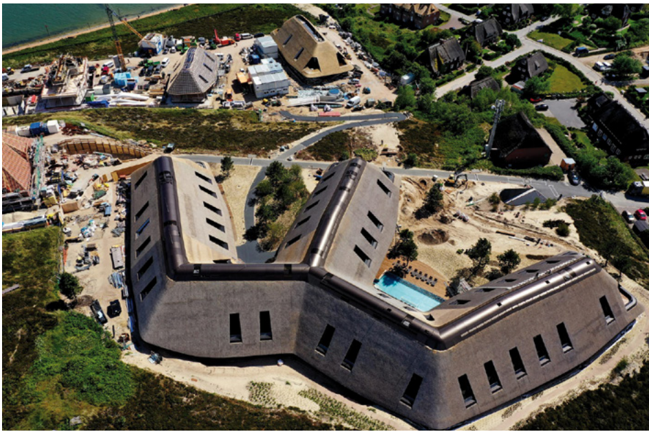
Fig. 21: Europe's largest thatched roof, Lanserhof on Sylt
