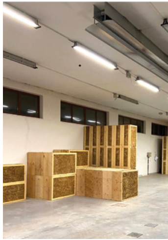
Fig. 18–20: Industrially prefabricated straw-insulated modules © Artem Ryzhkov, Life House Building
