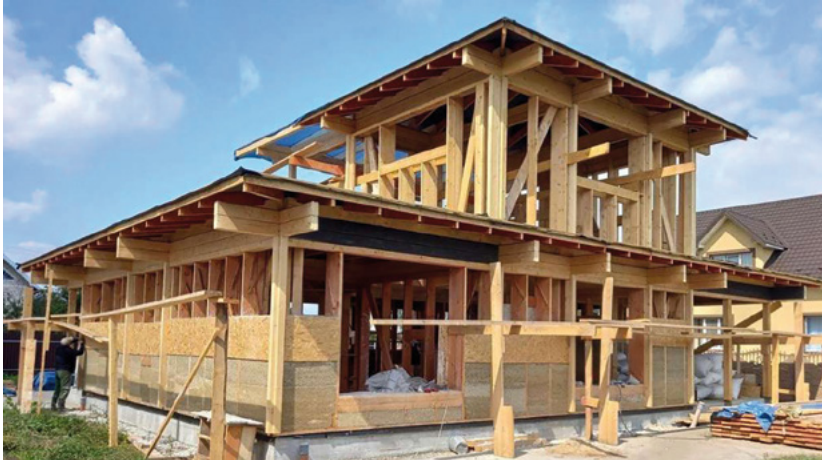
Fig. 16–18: Timber frame construction with hempcrete and hemp-lime infill in various construction phases © Hempire
